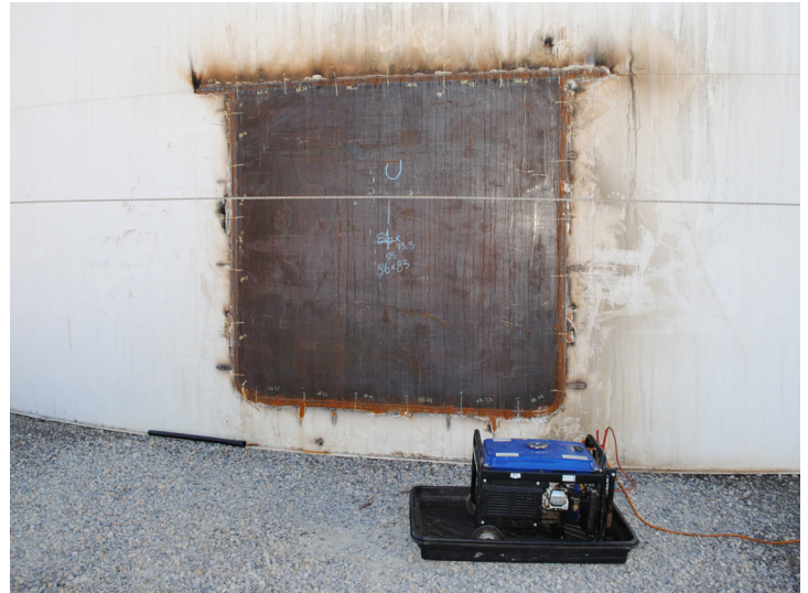
Aboveground storage tank repair prior to Zerios WES Temporary Coating.
